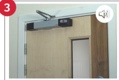
The Agrippa door closer recognises the fire alarm and automatically releases the door, protecting the building.
