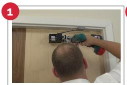
The Agrippa door closer is battery powered and wire-free. The device is installed at the top of the door.
